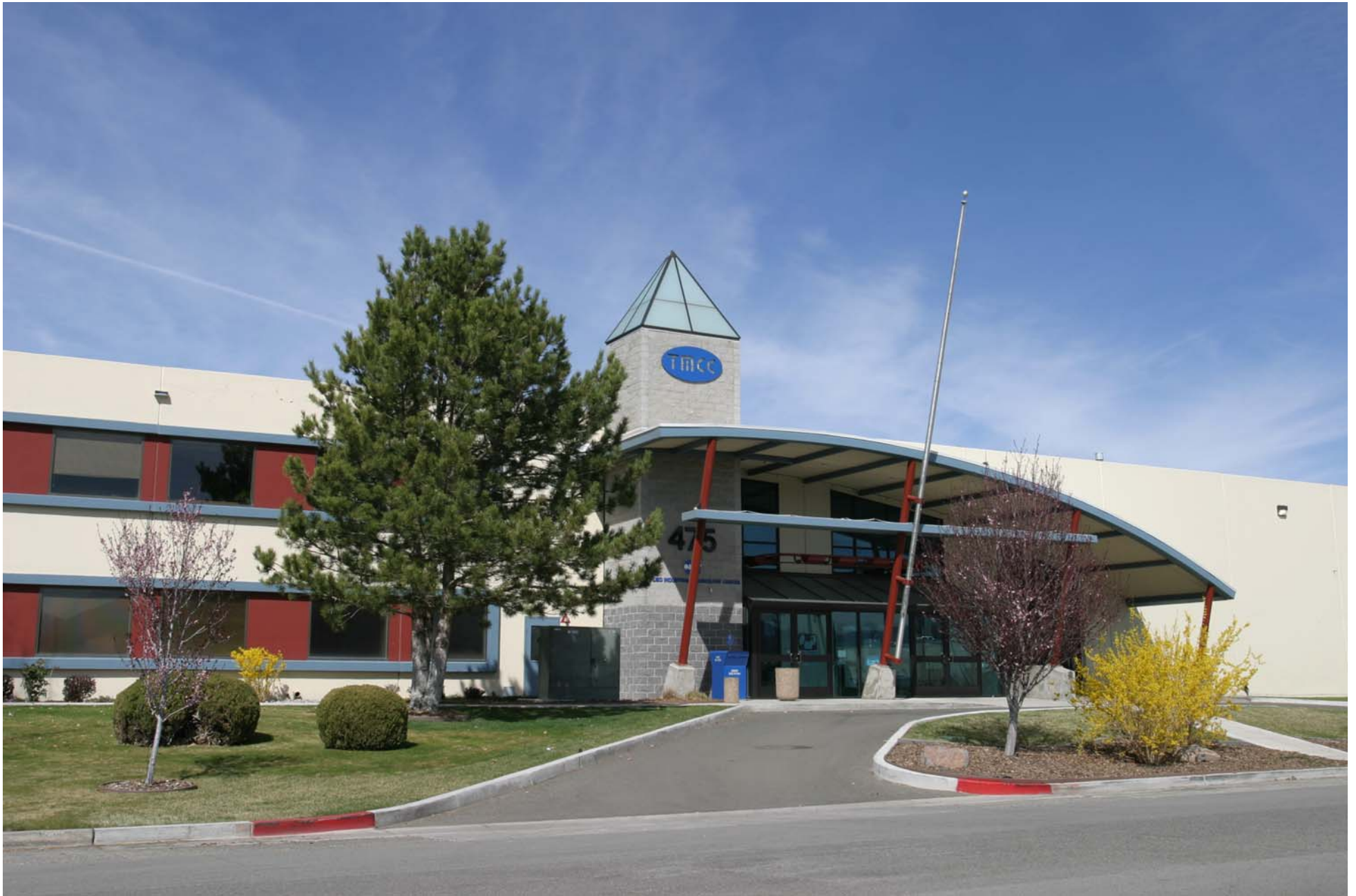
IGT-Applied Technology Center
